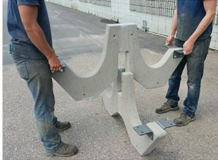
Attach eight seat brackets (#6) to leg (#5) to top and bottom interlocking leg with (#8) 3/8" x 5 1/2" hex Bolts, (#9) 3/8" locking hex nuts, and (#11) 3/8" flat washers. Note: use 3/8" flat washers on both sides of bracket. After installation of brackets on interlock legs, use brackets for lifting and assembly of Interlock legs.
