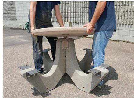
Mount table top and benches to installed brackets using (#10) neoprene pad and (#7) 3/8" x 1" hex flange bolts, four bolts per bench and top.
